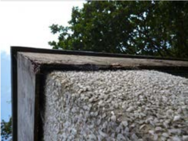
Target Note 7: Electricity sub-station with moderate bat roost potential relating to fascia board gaps.
